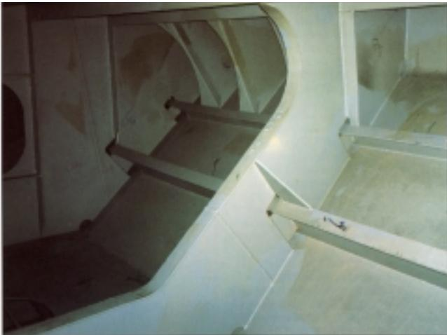
Inspection inside cargo tanks is much more difficult as it requires a lengthy process of washing, gas freeing and ventilation before they are safe to enter. Some double hull tankers have suffered rapid corrosion inside the cargo tanks, which are often not coated. **OCIMF has published a paper on this problem which appears to be far more serious than on single hull tankers. (Factors Influencing Accelerated Corrosion of Cargo Oil Tanks)**
